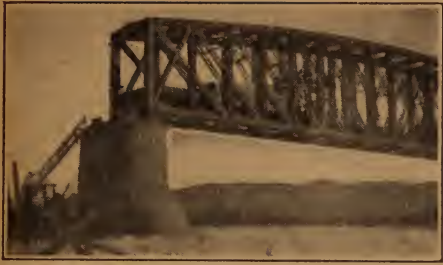
ONO BRIDGE, BLOWN UP BY BOLSHEVIKI.
